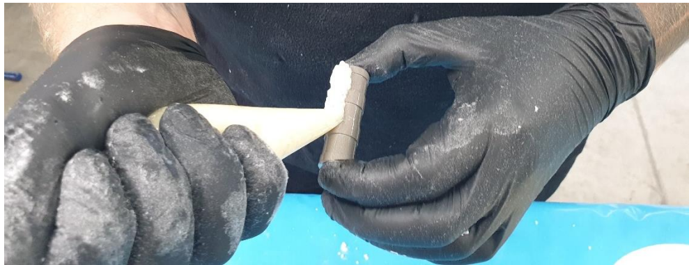
Fig. 20 – Applying HB20 to cylindrical surface of the bushing
