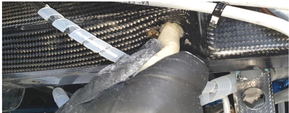
Fig. 21 – Applying HB20 into holes
